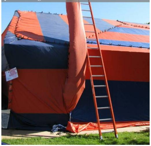
After completion of aeration, the fumigator must test the air in each room using the Interscan or SF-ExplorIR to confirm aeration of the fumigant before allowing reoccupancy of the building.
